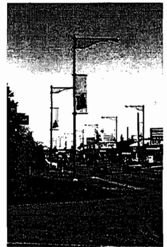
Gateway Boulevard Built View, August 1999 Repeating elements of the Gateway Blvd. lighting design in the Highway 2 Corridor will help build an integrated and consistent design standard between the Edmonton International Airport and Downtown Edmonton.
